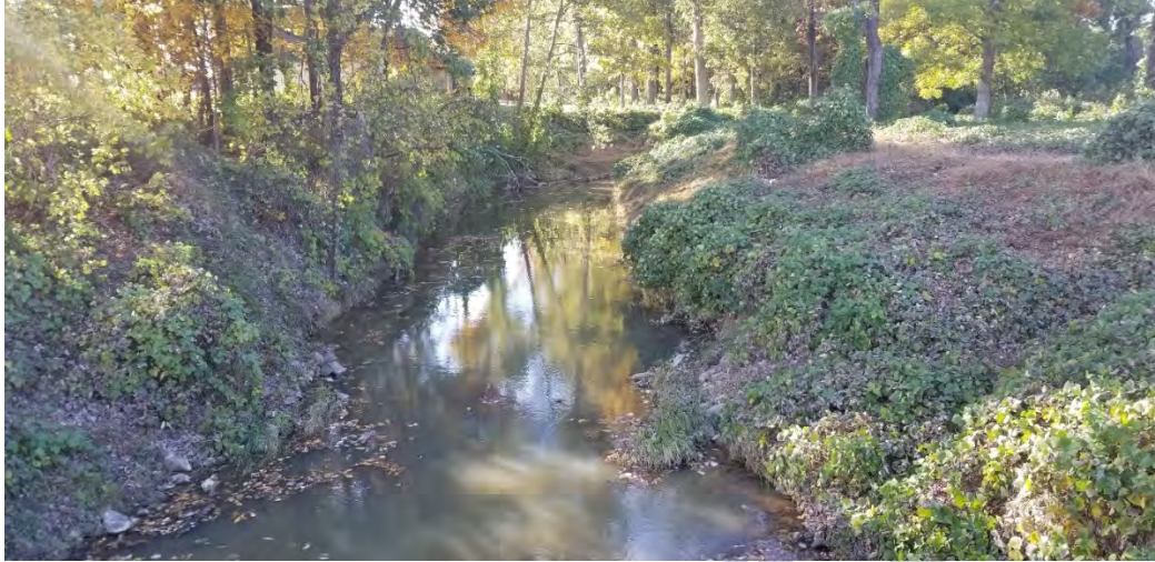
Figure 3. Nolehoe Creek-Malone Street culvert-looking upstream at stable channel
