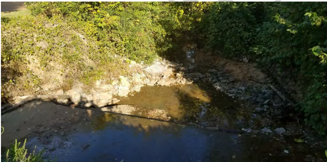
Figure 4. Nolehoe Creek-Malone Street culvert-looking downstream at channel degradation
