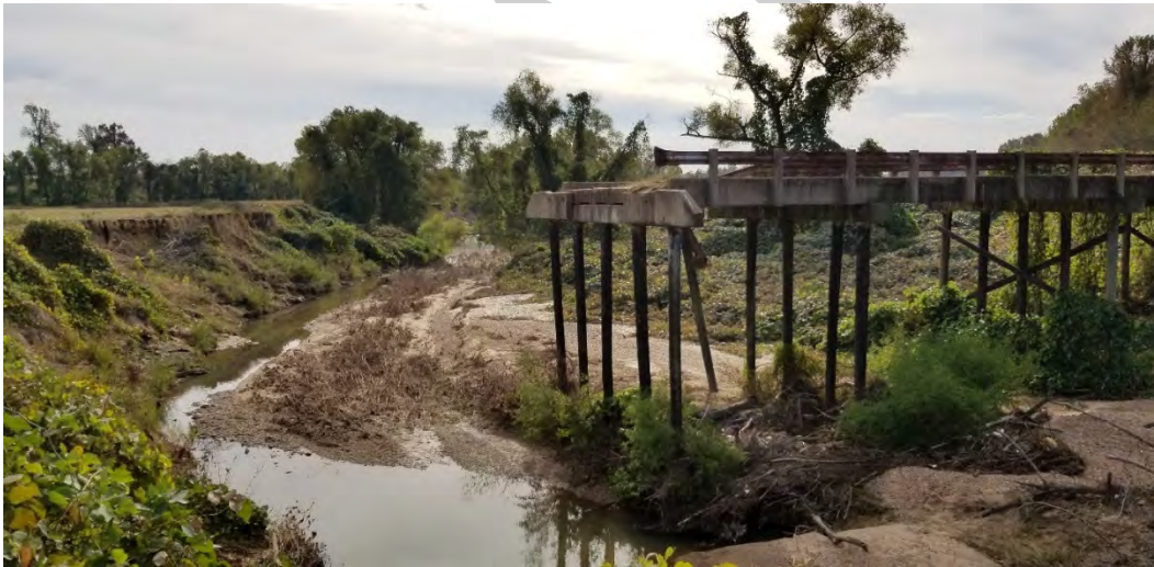
Figure 28. Nolehoe Creek-Sand Ridge Road Bridge failure site (left bank)
